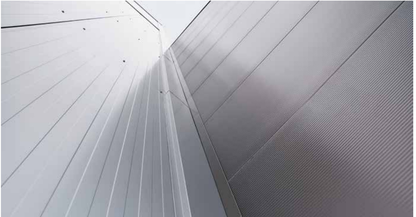
30m tall deep-freeze high-bay storage warehouse
